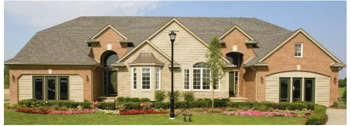
Stoneridge at Heritage Village by Sable Homes.
